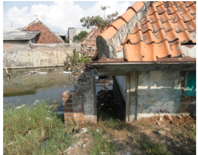
Fig. 5. Permanently abandoned homes in the Kemijen area (2013).
