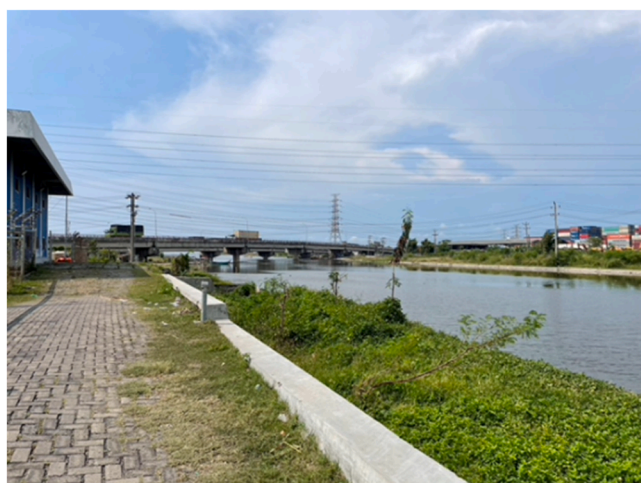
Fig. 9. Banger river and river embankment with pumping station on the left (2022).
