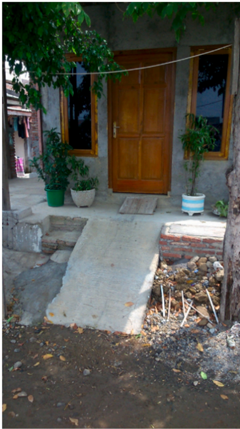
Fig. 3. Ground floor is being given up and filled with stones to compensate for land subsidence and tidal floods in Kemijen neighborhood (2013).
